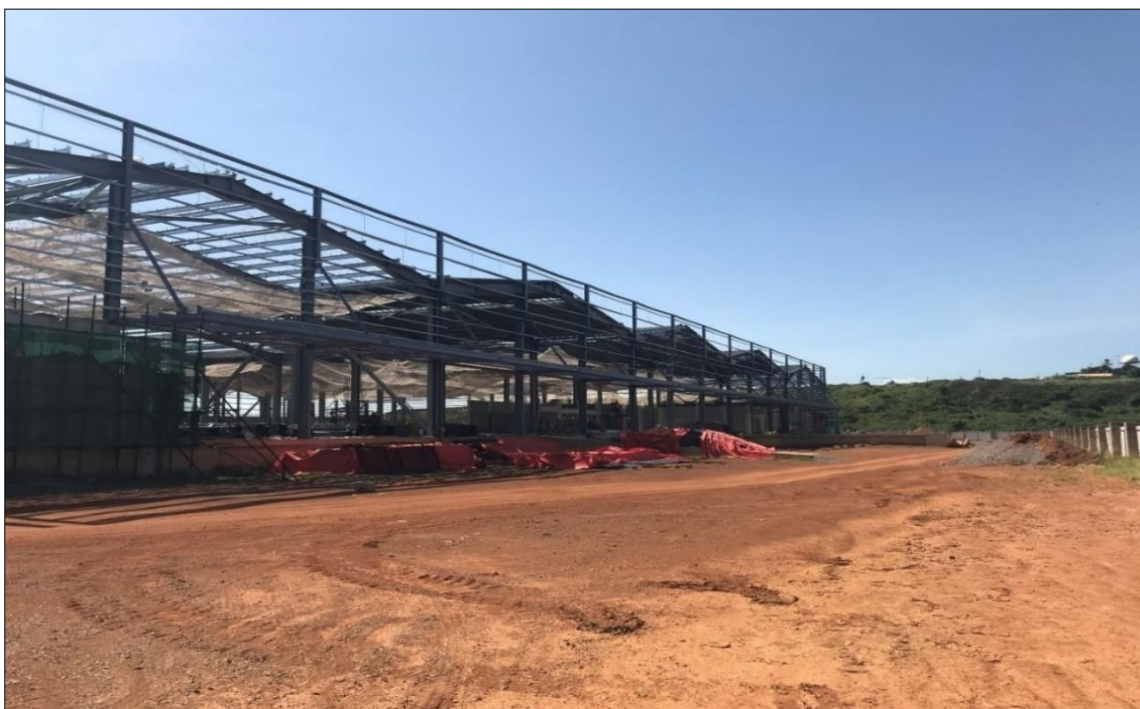
Figure 16: New Cargo Facility Construction (March 2019)
