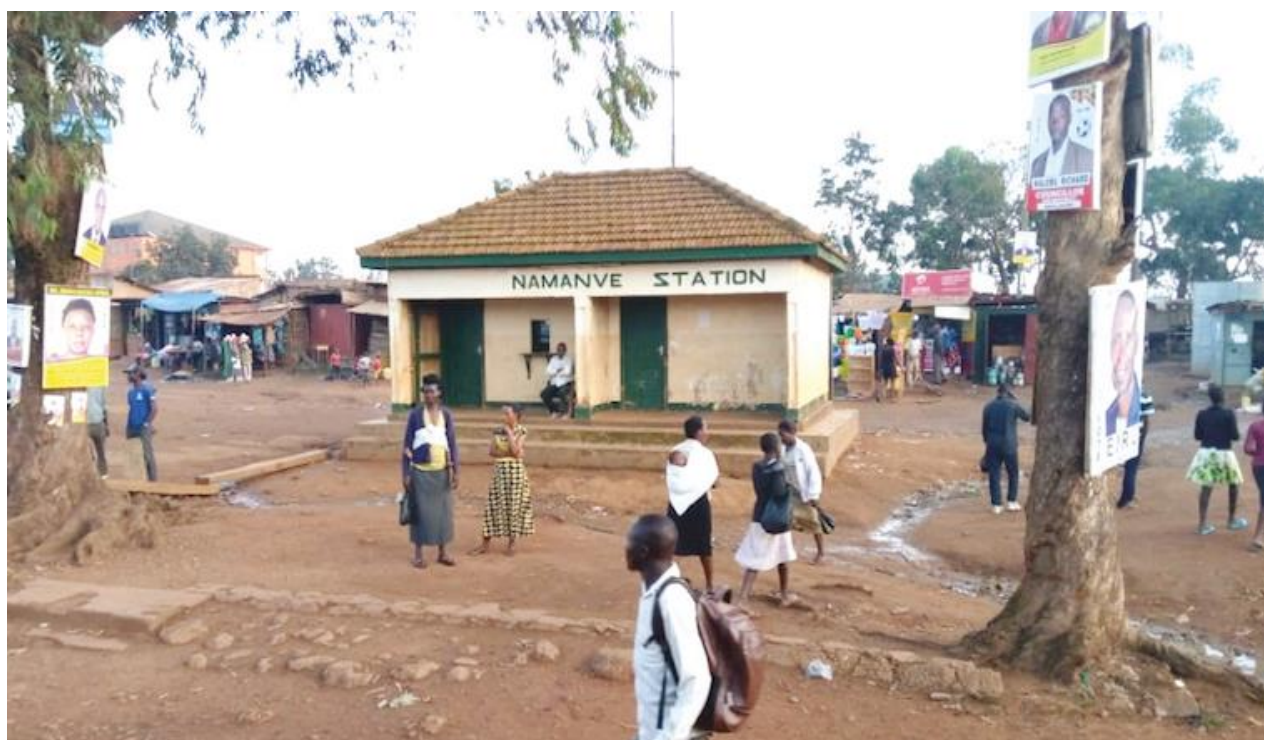
Figure 7: Dilapidated Namanve passenger railway station in Mukono district
